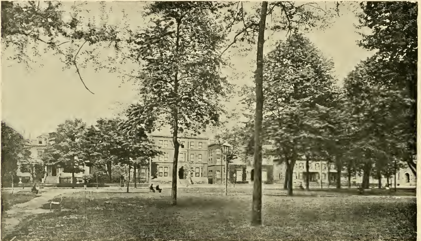
VIEW ON WASHINGTON PARK AND WASHINGTON STREET.
